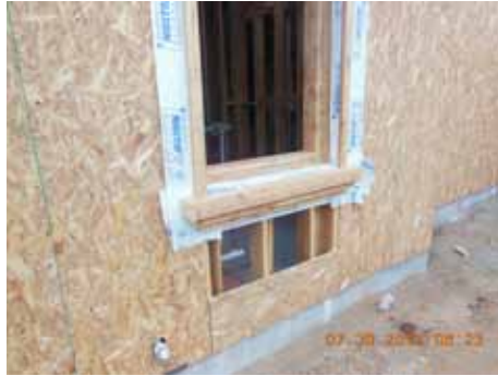
1. Exterior recessed framing condition
