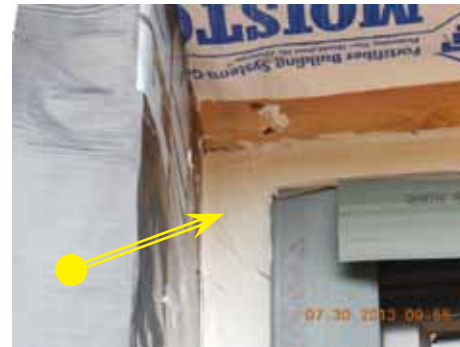
17. Apply sealant on top of nailing fin and butter flat
