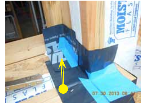
7. GS 100 B flashing corner set in place
