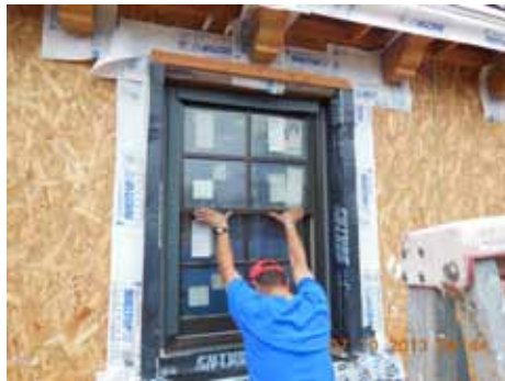
15. Apply side layers of window flashing (Future Flash) and set the window in place.
