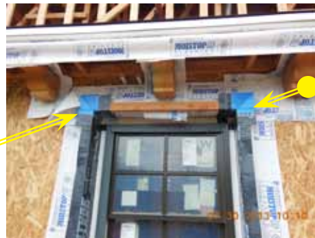
19 & 20. Apply top GS 106 A flashing corners into the wet sealant as shown. Wet sealant at top corners (not shown).
