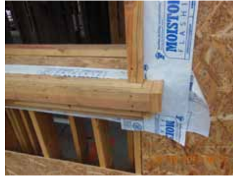
2. Exterior recessed framing condition
