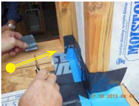
8. Trim GS 100 B corner @ framing sill
