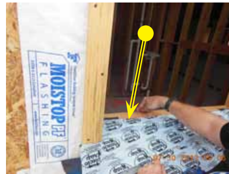
10. Protecto Wrap layered on to framing sill as shown
