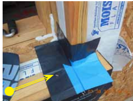
5. GS 106 A flashing corner set in place
