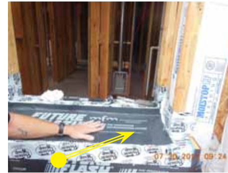
14. Apply lower course of window flashing (Future Flash)
