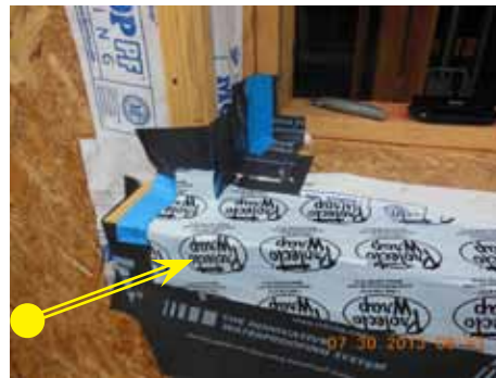
9. Begin to apply Protecto Wrap SAF flashing; layered to overlap minimum of 4 inches.
