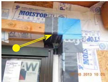
19 & 20. Apply top GS 106 A flashing corners into the wet sealant as shown. Wet sealant at top corners (not shown).
