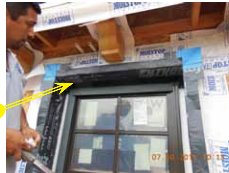
21. Apply top window flashing (Future Flash)
