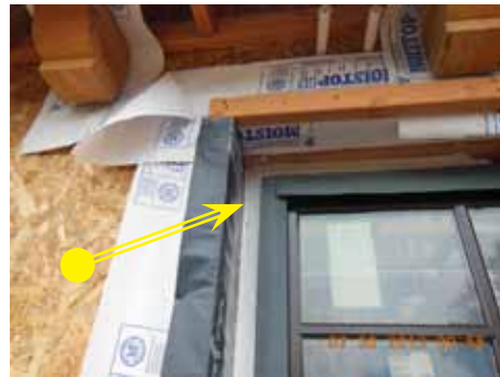
16. Apply sealant on top of nailing fin and butter flat
